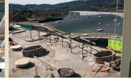
One-way truss system (left) and rolling green roof construction (right) at Palomar Medical Center West
